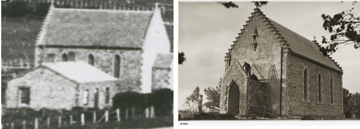
Figure 2: St John the Evangelist Church. Left 1898 and right being demolished in 1936. Both photos courtesy State Library. Catalogue numbers B17124 and B9495.
